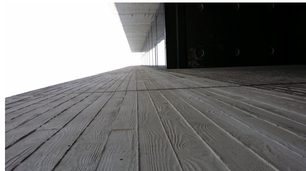
Got Concrete? (Existing Long Beach City Hall)
